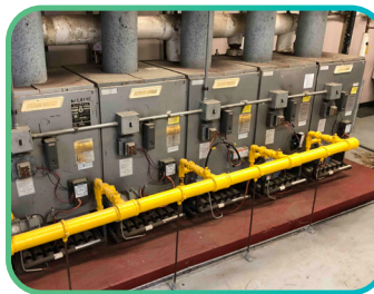
Before (left) and after (right) RLE upgraded an outdated boiler system with a new, energy-efficient system.
